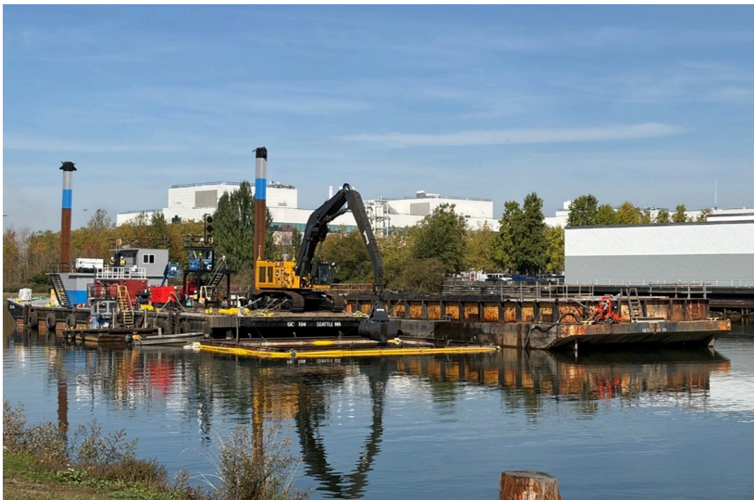
Dredging equipment, mounted on a barge, removes contaminated sediment at sediment management area 16. (King County, October 2026)
