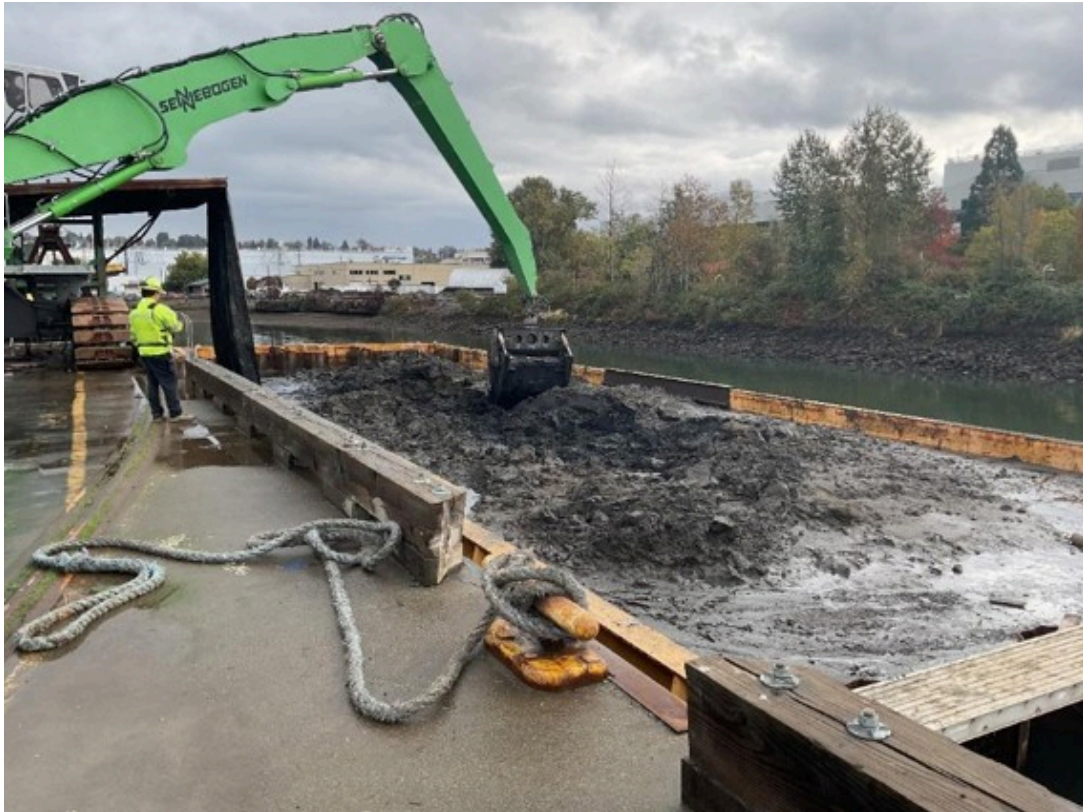
Removing (or offloading) contaminated sediment from barge at Duwamish Reload Facility. This facility is where contaminated sediment is removed from each barge and loaded into rail cars. It is then transported and disposed at a permitted landfill. Photo Credit: Geosyntec
