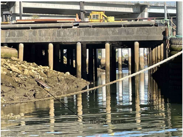
PIER (LOOKING UPSTREAM)
