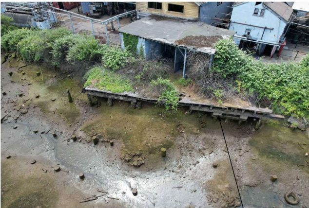
BUILDING PHOTO SCALE: NONE 2
