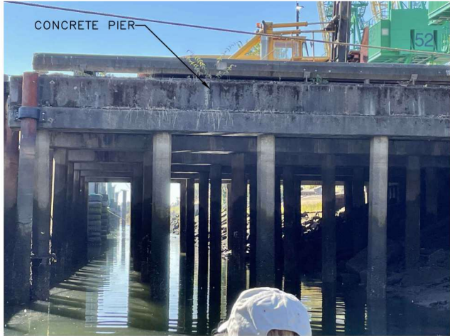
PIER (LOOKING DOWNSTREAM)
