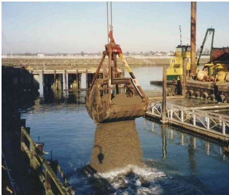
Controlled bucket placement
