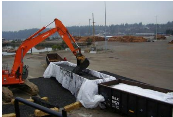
Loading of sediment into lined containers
