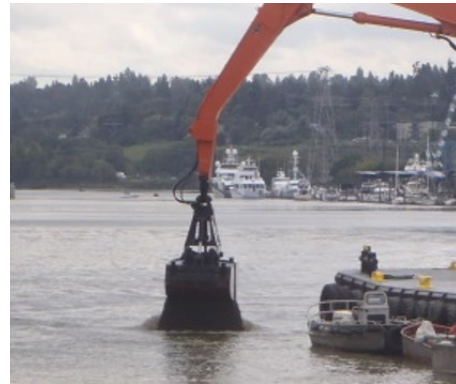
Controlled bucket placement
