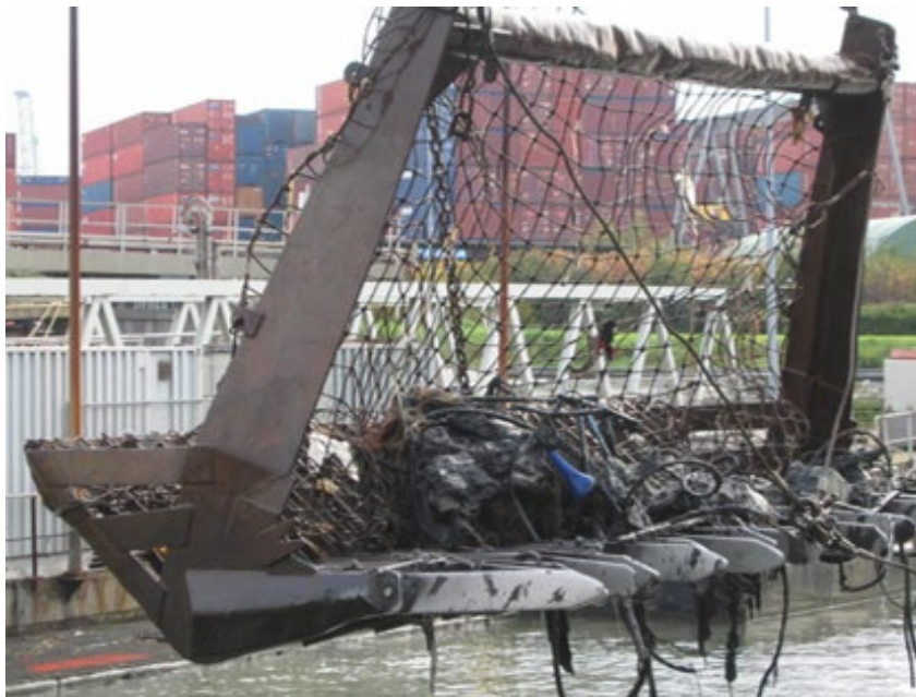
Exhibit 10-1 Debris Removal Prior to Dredging
